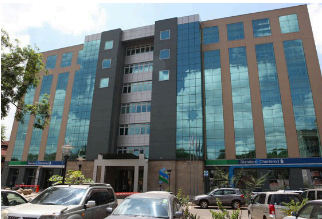
Structural Assessments at SCB Headquarters Building, Westlands road, Nairobi.
