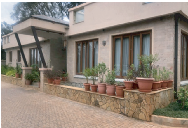
Design and Construction supervision of double storeyed residential building at Lavington. Associated structures such as guard house, machine storage house, DSQ, generator house, retaining boundary walls and drainage systems formed the project scope.
