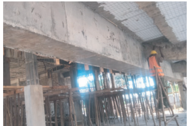
Adoption of post tension (PT) Technology for reinforced beam (26m span) at CPK Church, Kericho
