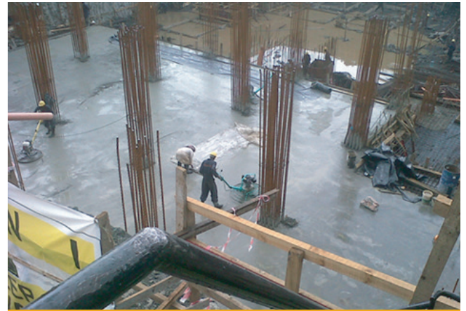
Power floating concrete Basement floor, Upper Hill Office Building
