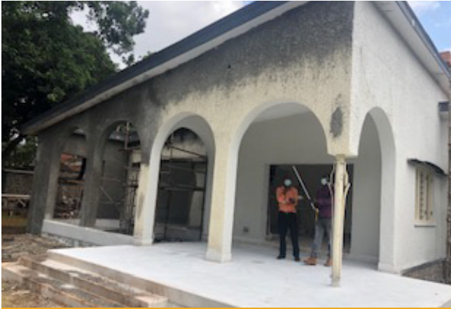
Office Extensions, Riverside Drive – Assessment, Design & Construction
