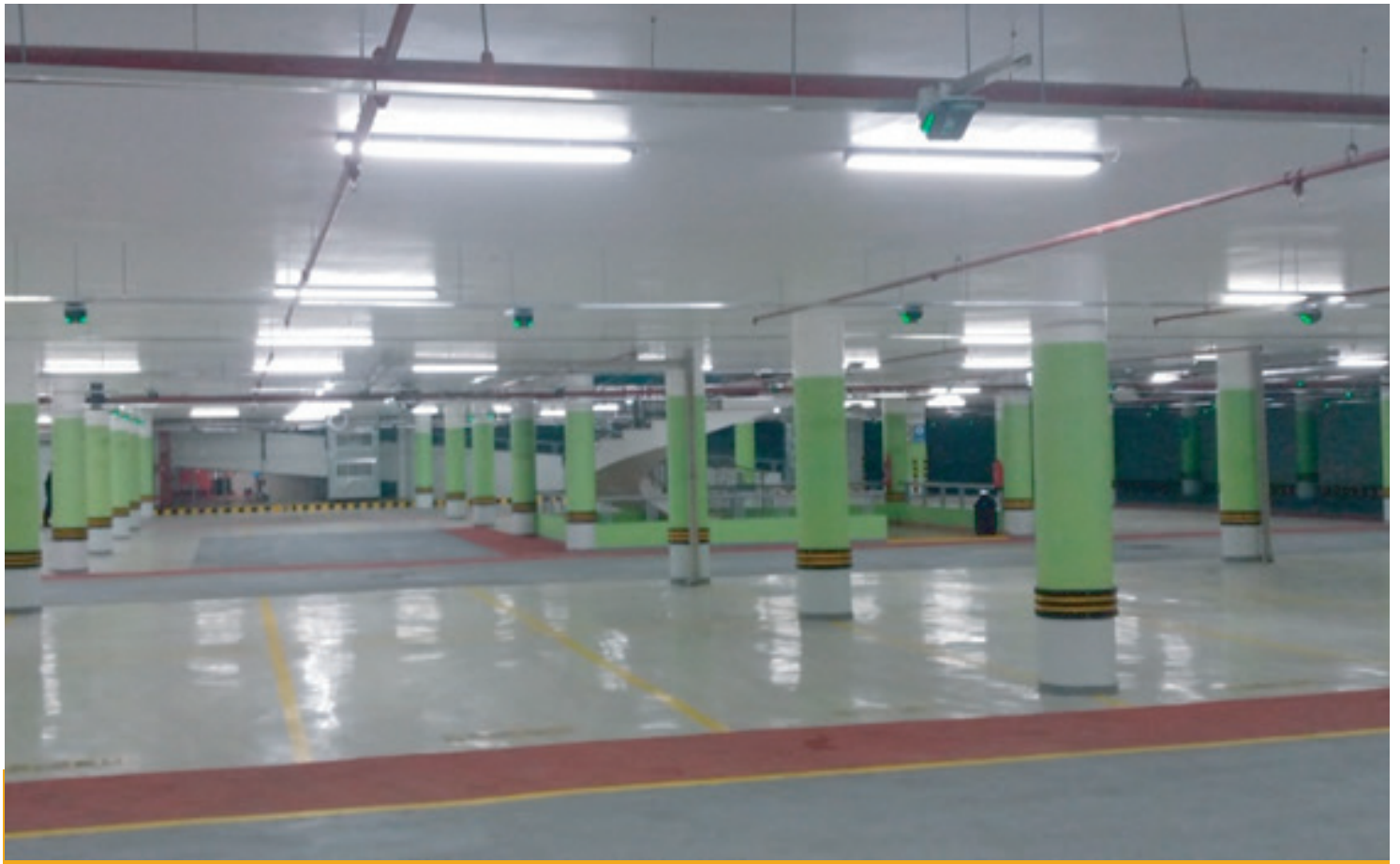
Construction supervision of a PT construction technology at Holy Basilica Underground Parking Silo
