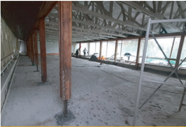
Structural Assessment for installation of new suspended floor and renovation construction at Air Kenya Offices, Wilson Airport, Nairobi.
