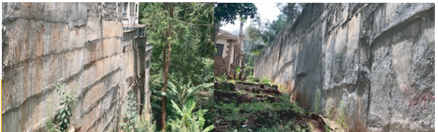
Retaining Wall Assessment, Peponi Road For Aga Khan Foundation
