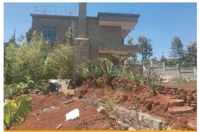
Design and Construction supervision of double storeyed residential building at Tigoni. Engineering solutions were implemented for stabilizing of steep slopes for garden landscape and stormwater management.
