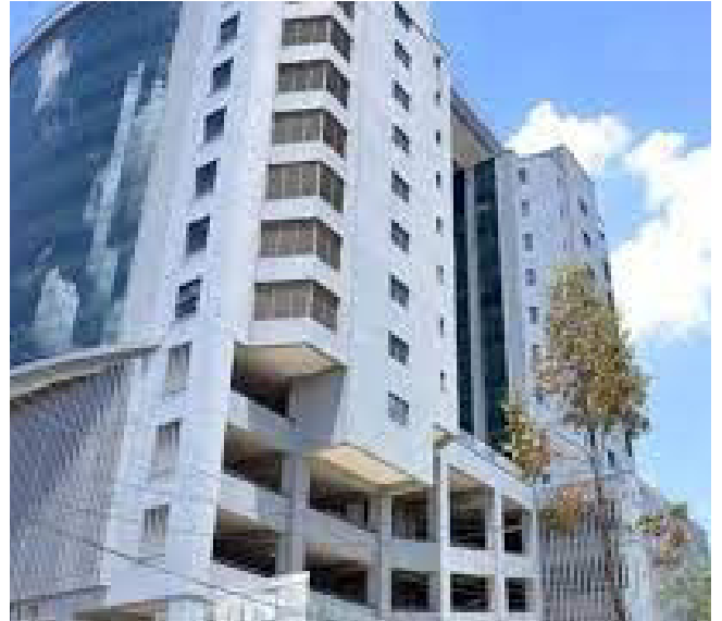
Jamii Towers With Rooftop Helipad, Upper Hill, Nairobi
