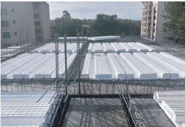
Design and Construction supervision of EPS concrete suspended floors for residential apartments at Thindigua, Kiambu road.
