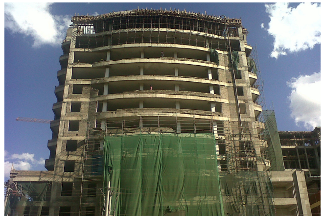
13 Storey Jamii Towers Office Building with 2 Basement floors and Roof Helipad at Upper hill, Nairobi
