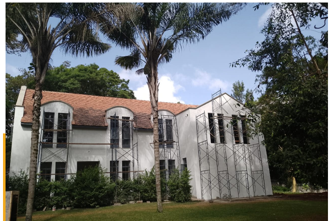
Residential House, Karen – Engineering Design & Construction
