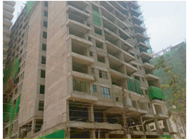
Residential apartments construction - concrete volume assessment. Gazebo apartment, 3rd Parklands AV
