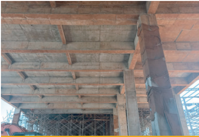
15M Span Post-Tension (PT) reinforced concrete Shallow beams Forming part of the slab deck, a solution to omit deep beams and create sufficient headroom at the Temple in Parklands.
