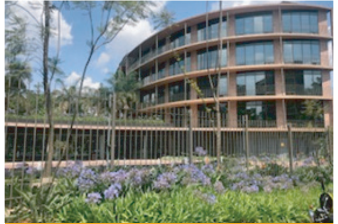
Structural Assessment for PDM, Vienna Court, State House Rd.
